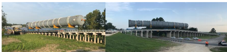
Semi Permanent Levee Crossing – YCI - Donaldsonville LA
