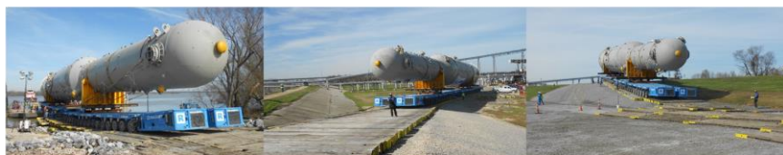
Matted Earth filling Levee Crossing – Valero - Donaldsonville LA
